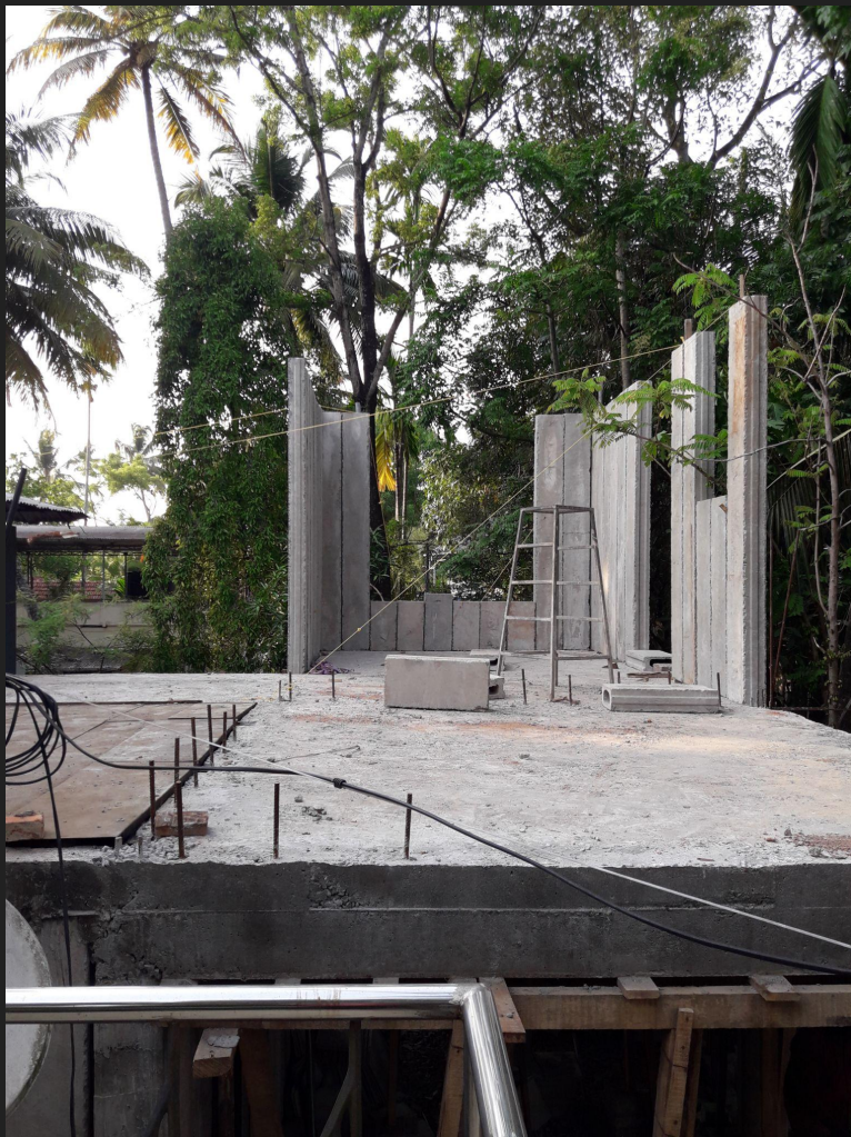
20.ERECTING WALLS ON 1ST FLOOR
